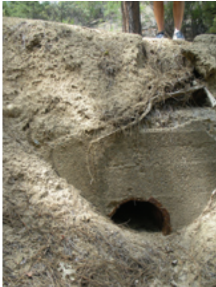
MUD IN WATER: Forest road culvert delivering sediment to waterways.
